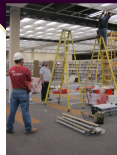
Library renovations began May 31, 2011
