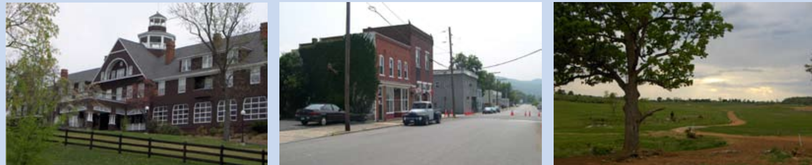
HISTORIC PRESERVATION AND ADAPTIVE REUSE (FAIRFAX HALL, RESERVOIR STREET) REDEVELOPMENT AREA (COMMERCE AVENUE) LOCAL LANDSCAPE AND OPEN SPACE
