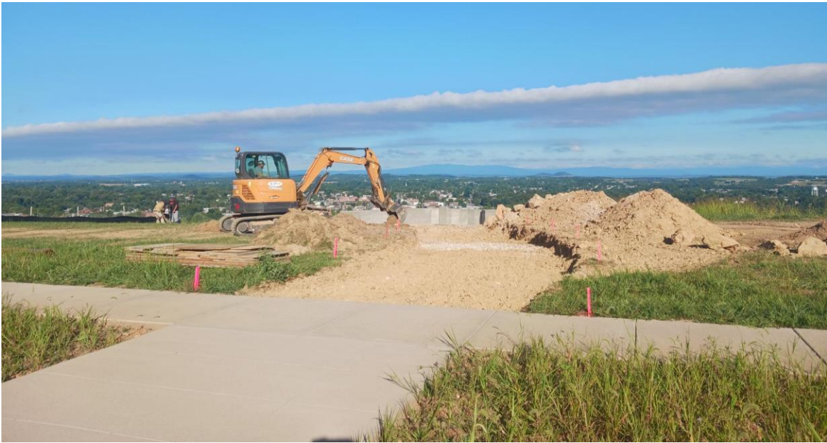
Grading of walkway to large overlook.
